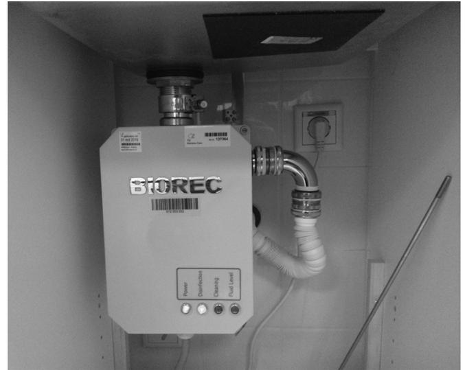
**Figure 1.** The self-disinfecting Medizinische Hygiene-Siphon BIOREC (MoveoMed, Dresden, Germany).
